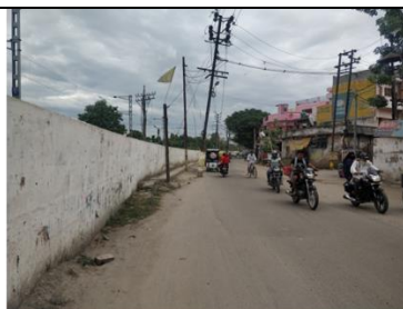
P1 Road Condition
