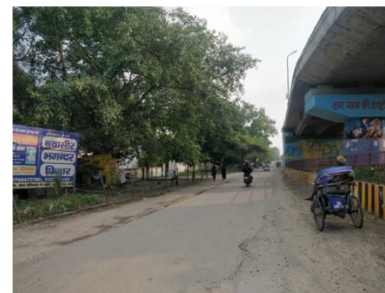
Road below Flyover
